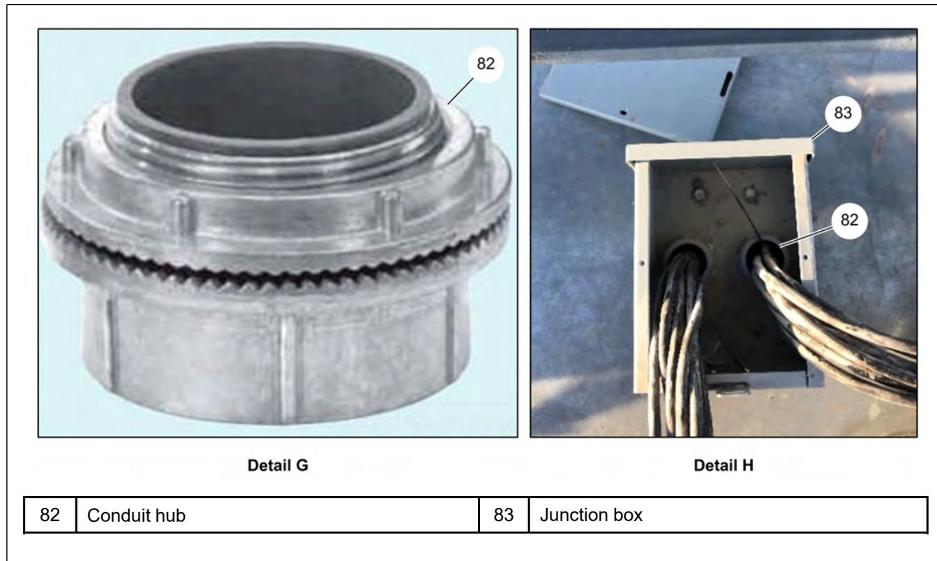
Figure 5-21 Routing the Mux Box interconnect cable through side cable gland
