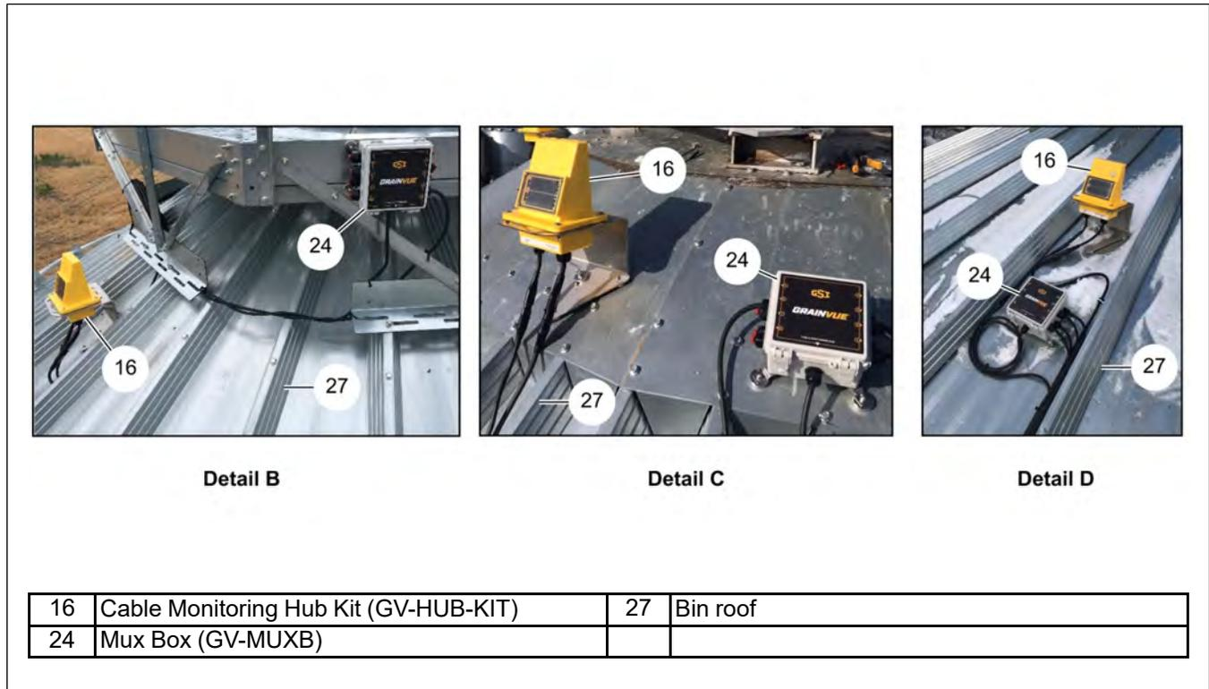
4. Route, secure, and connect the interconnect cable (20) from the Mux Box (24) to the port labeled Cables on the Cable Monitoring Hub (16) (push the connectors together until the tab clicks and locks in place).
