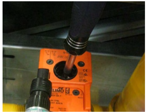
Image 7 – Setting valve to 0% open
