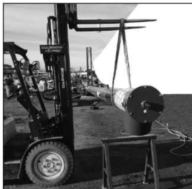
FIG. 3-17. Lifting the Discharge End of Tube
