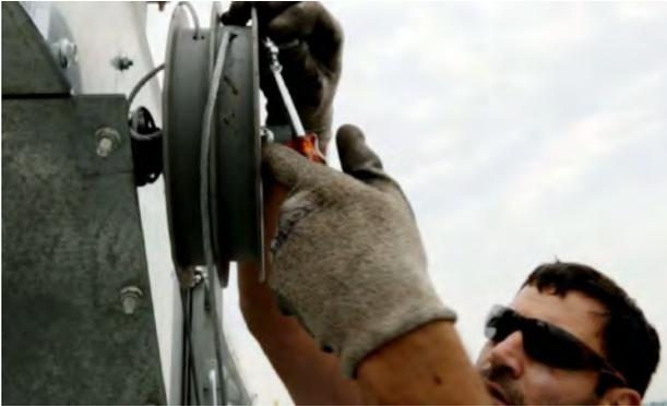
**Image 8 – Clamping cables to top pulley**
