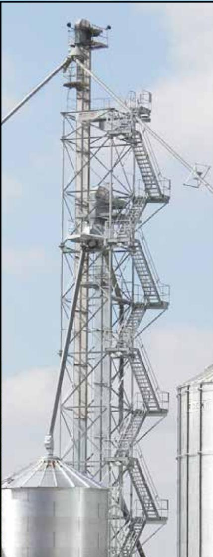
Service Stairway and Custom Walkways to Varying Height Elevator Platforms
