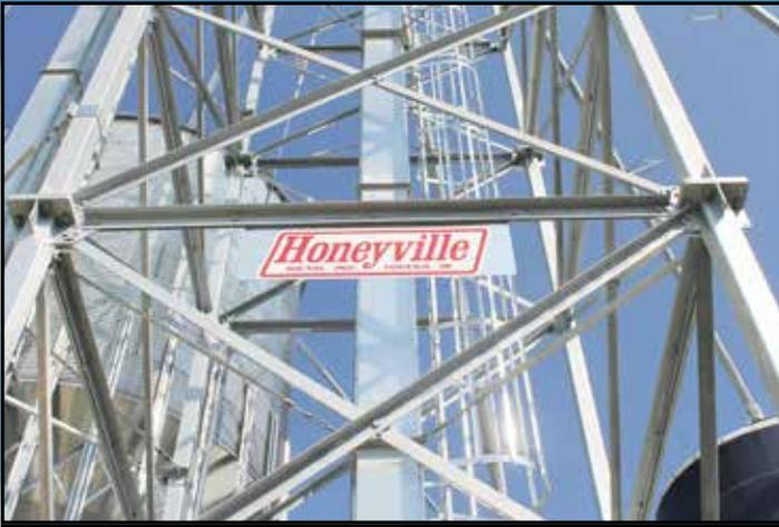
125' Tower: Dry Elevator Inside, Wet Elevator Outside and Service Ladder on Elevator
