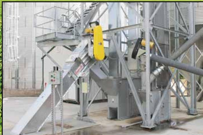
V-Bracing for Conveyor Access to Elevator Boot
