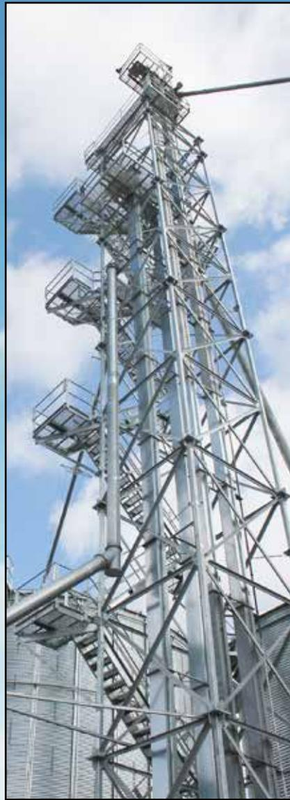
105' Tower: Dry and Wet Elevators Inside Tower and Service Stairway Option
