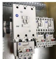
Contactors & Overloads
