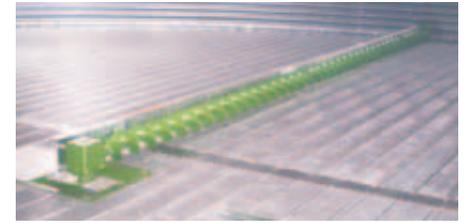
**Sukup Hawk Cut™ Bin Floors and Z-Post or Super Supports** provide a solid base for your grain. Sukup Hawk Cut™ floors are extra-strong since no steel is removed while creating the open areas in the planks.
