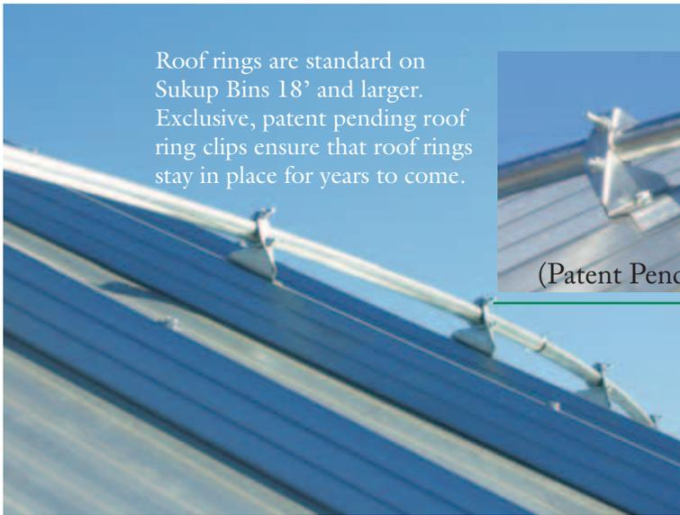
Roof rings are standard on Sukup Bins 18’ and larger. Exclusive, patent pending roof ring clips ensure that roof rings stay in place for years to come.
